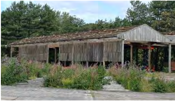
Photograph 3: Building (B4) on-site (06.08.2025).
