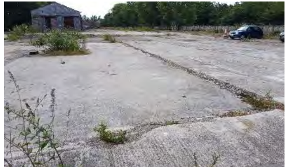
Photograph 2: Hardstanding with scattered buddleia scrub (06.08.2025).
