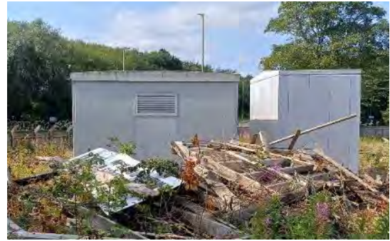
Photograph 4: Building (B7) on-site (06.08.2025).
